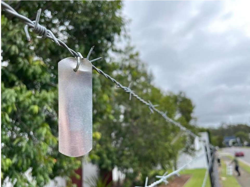
Figure 2: Recommended tag installed on barbed wire fence
